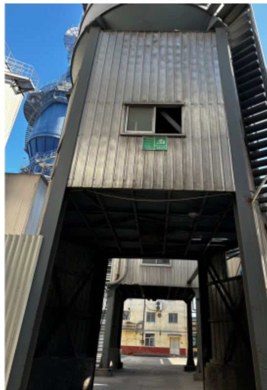
ts003 粉煤灰储存库
